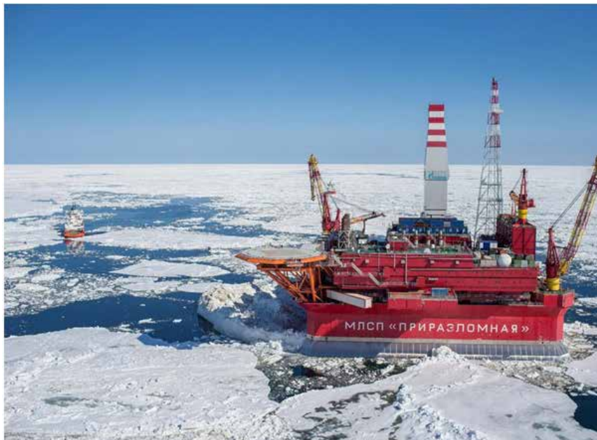
Fig description & source: The Prirazlomnaya platform is the first Russian project for developing the Arctic shelf. (Humpert et al., 2011)
